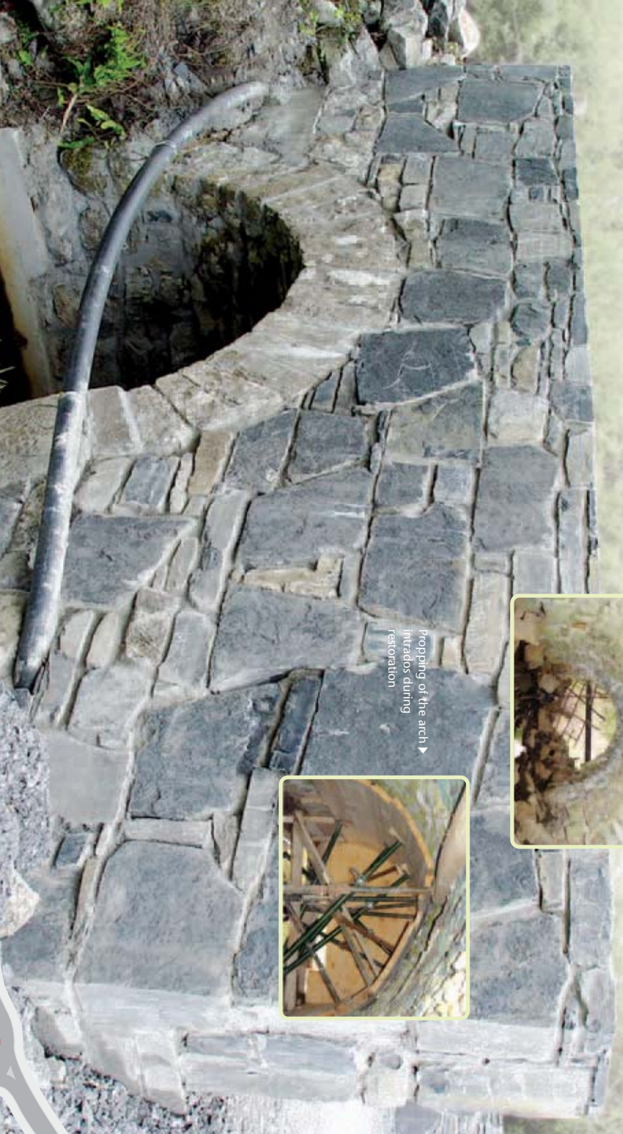
▶ New foundations, rebuilt and pointed abutments.
