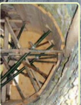
▶ Propping of the arch intrados during restoration
